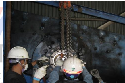
▷ Vibrating Screen Bearing 교체
